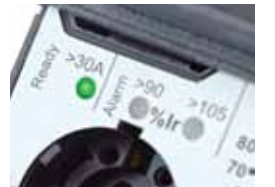
The green "Ready" LED flashes to show that all is well.
